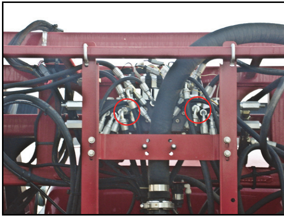
FIGURE 11. Left and Right Down Hoses Installed
