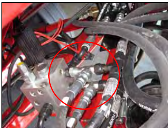
FIGURE 3. Pressure and Tank Hoses Installed
