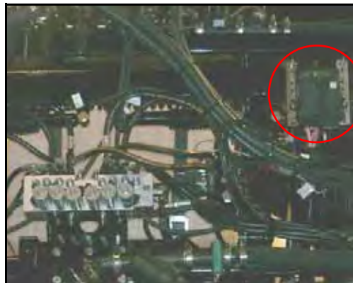
FIGURE 11. UltraGlide AutoBoom Node Installed
