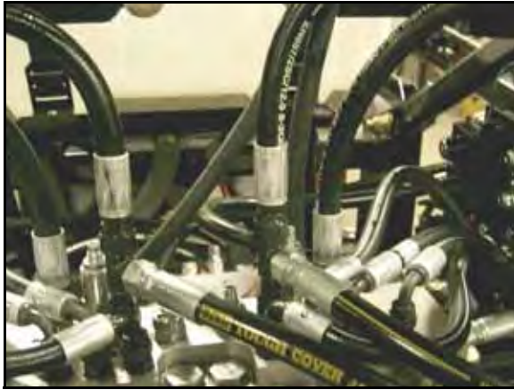
FIGURE 4. Left and Right Cylinder Hoses Installed
