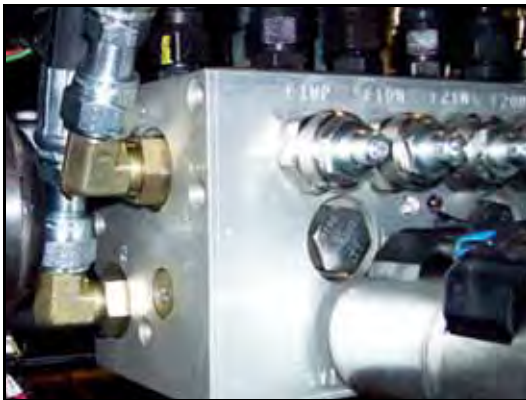
FIGURE 3. Pressure and Tank Hoses Installed
