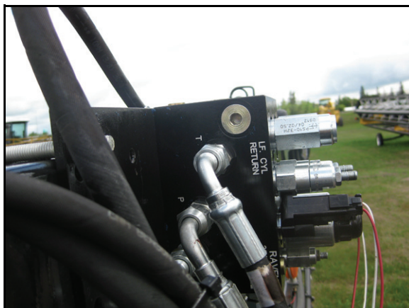
FIGURE 5. Pressure and Tank Lines Installed
