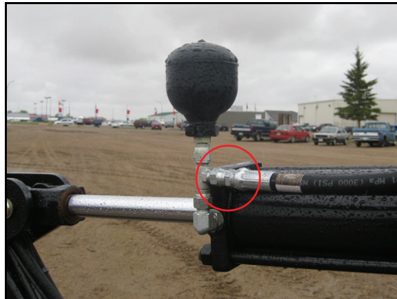
FIGURE 13. Hydraulic Hoses Installed on Machine's Cylinders
