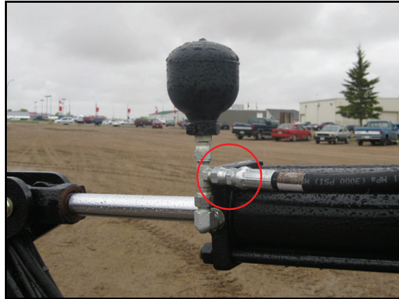
FIGURE 7. Hydraulic Hoses Installed on Machine's Cylinders
