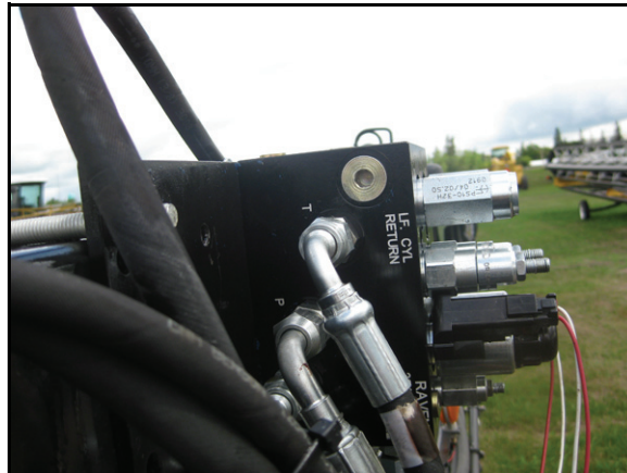
FIGURE 11. Pressure and Tank Lines Installed
