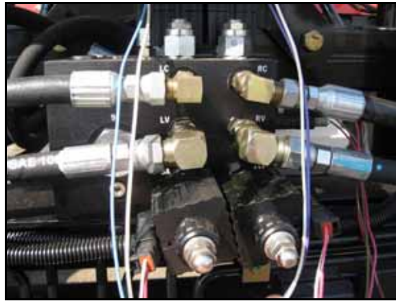
FIGURE 6. Cylinder Hoses Installed on the AutoBoom Valve
