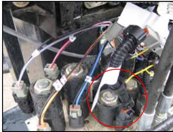
FIGURE 16. Machine's Left and Right Tilt Boom Function Coils
