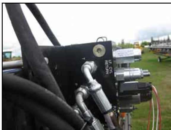
FIGURE 11. Pressure and Tank Lines Installed
