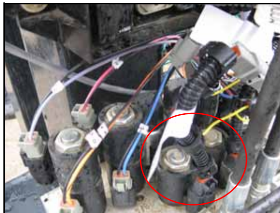
FIGURE 9. Machine's Left and Right Tilt Boom Function Coils
