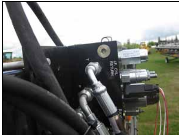
FIGURE 5. Pressure and Tank Lines Installed
