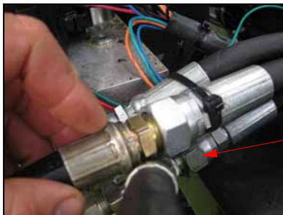
FIGURE 4. Extension Hose Installed on Machine's Pressure Hose
