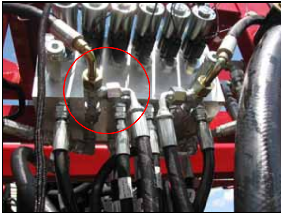
FIGURE 5. Left Cylinder Hose Installed
