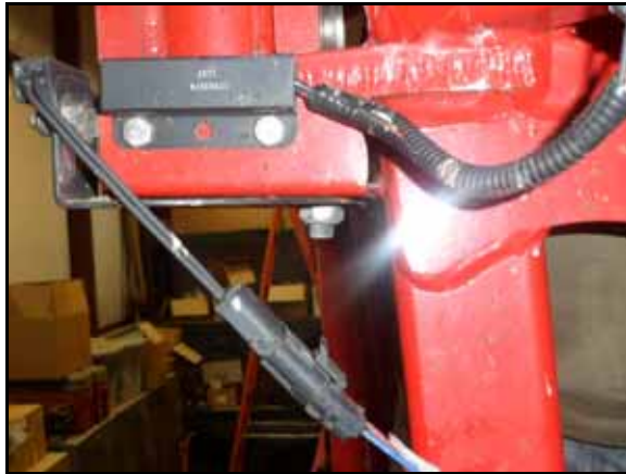
FIGURE 7. Extension Cable Installed on Sensor
