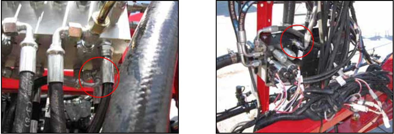
FIGURE 7. Right Down Hose Installed
