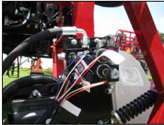
FIGURE 2. AutoBoom Harness Connected to Valve
