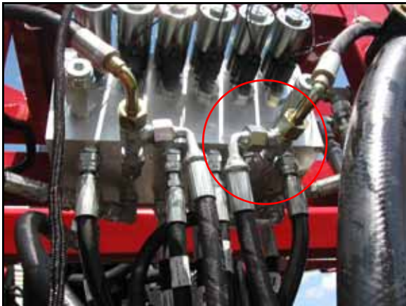
FIGURE 4. Right Cylinder Hose Installed
