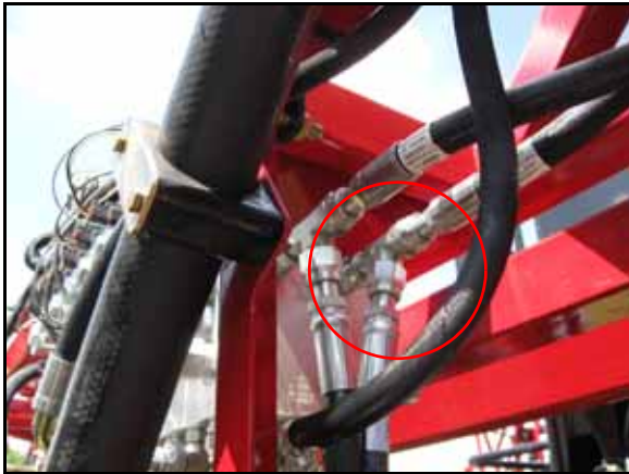
FIGURE 3. Tank Hose Installed
