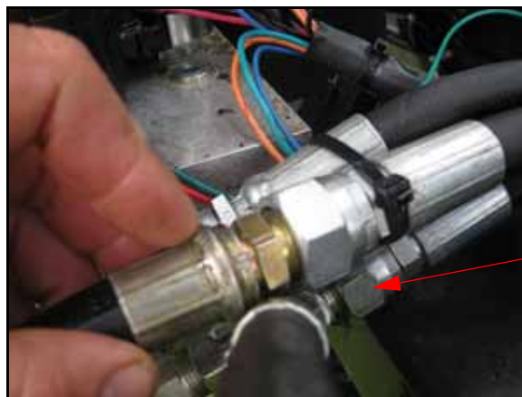
FIGURE 4. Extension Hose Installed on Machine's Pressure Hose
