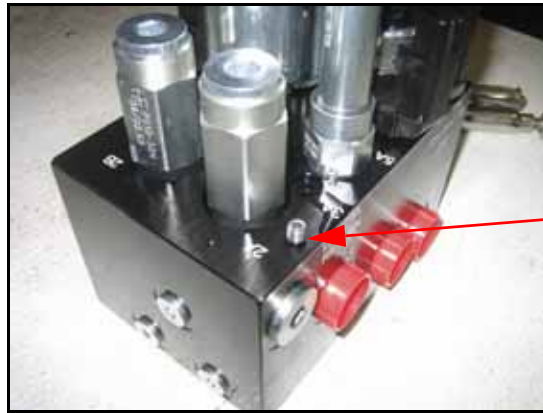
FIGURE 5. Orifice Fitting Removed from the AutoBoom Valve
