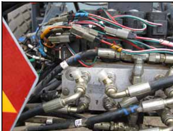
FIGURE 8. Machine's Down Hoses Installed on Tee Fittings
