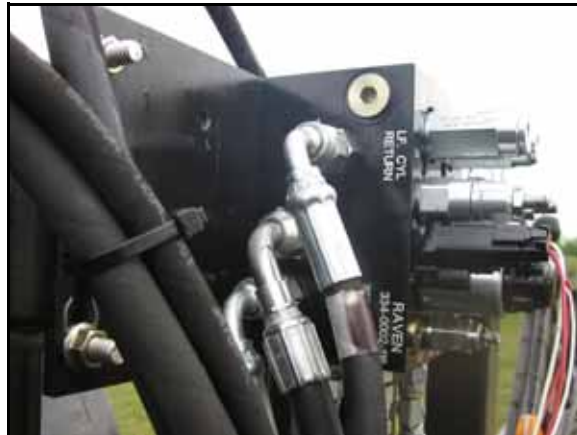
FIGURE 5. Pressure and Tank Lines Installed
