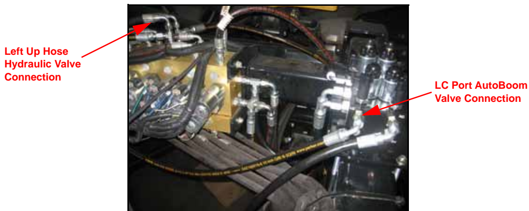
FIGURE 11. Left Cylinder Up Hoses Installed
