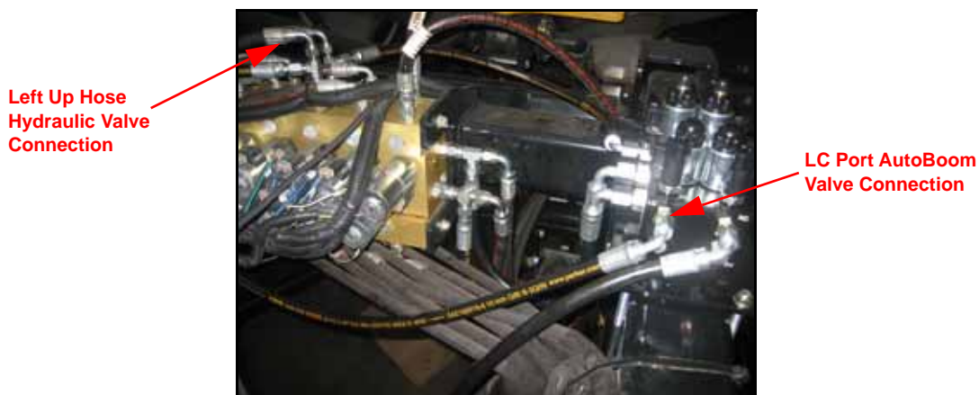
FIGURE 5. Left Cylinder Up Hoses Installed
