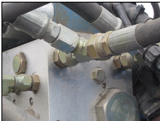
FIGURE 5. Tank Hose Installed
