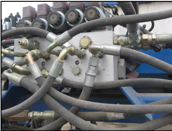
FIGURE 12. Cylinder Hoses Installed
