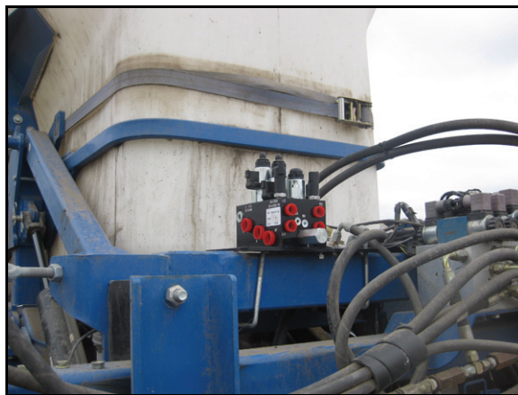
FIGURE 3. AutoBoom Valve Mounting on the Machine
