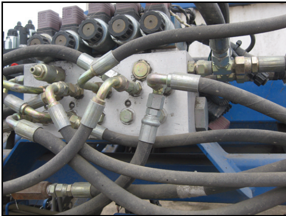
FIGURE 6. Cylinder Hoses Installed
