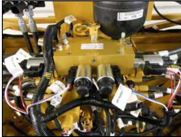
FIGURE 12. Valve Harness Installed on AutoBoom Valve
