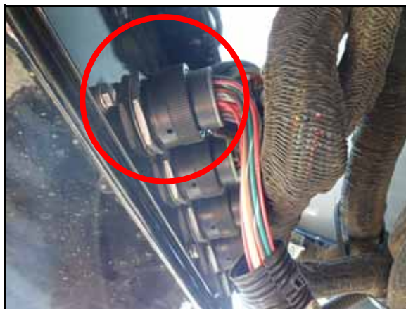
FIGURE 13. Valve Harness Installed on Bulkhead
