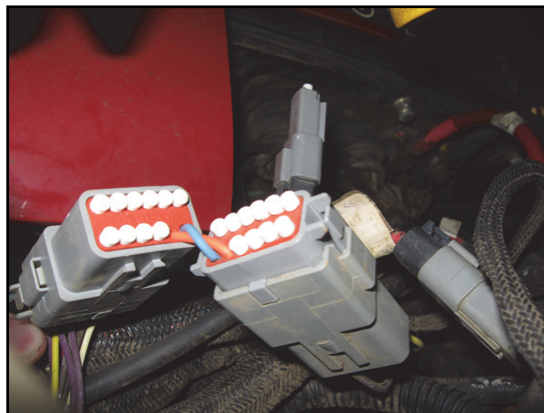
FIGURE 10. FIGURE 7. Fence Row Adapter Cable Installed
