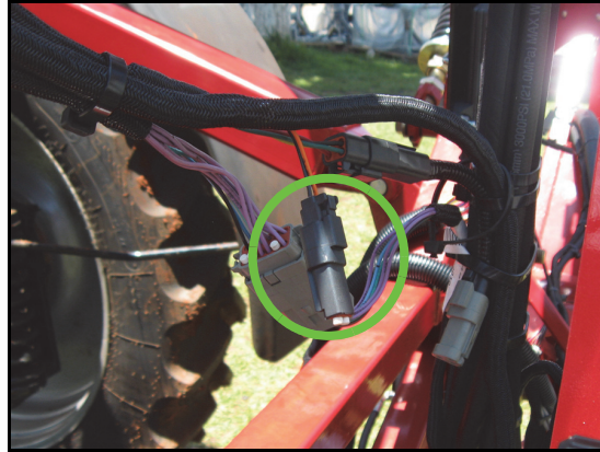
FIGURE 7. Machine's Existing Power Connection
