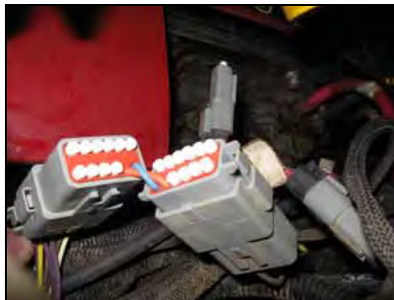
FIGURE 7. Fence Row Adapter Cable Installed
