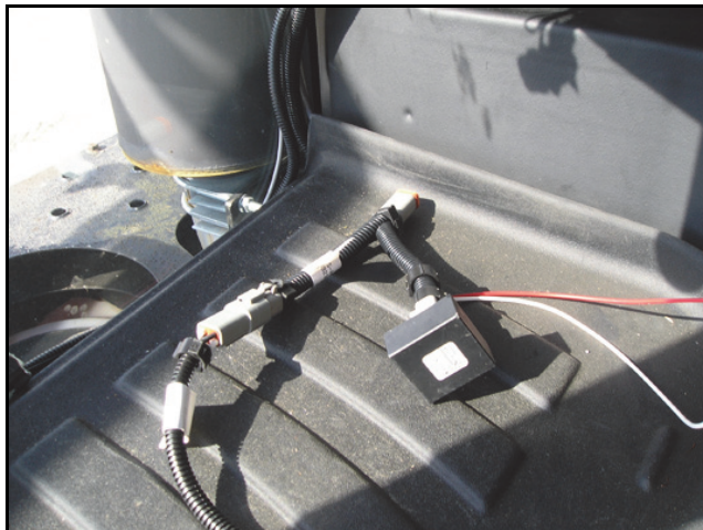
FIGURE 3. Power Tee Cable Connections
