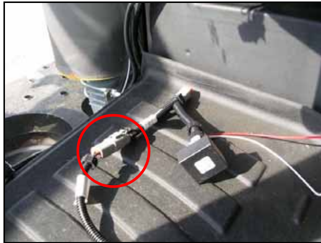
FIGURE 2. Field Computer Cable Connection
