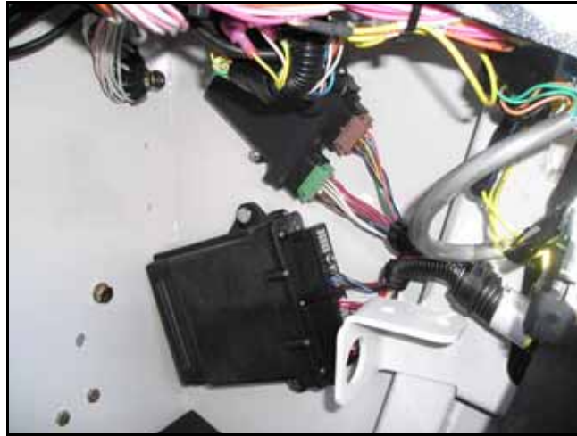
FIGURE 4. AccuBoom Node Installed
