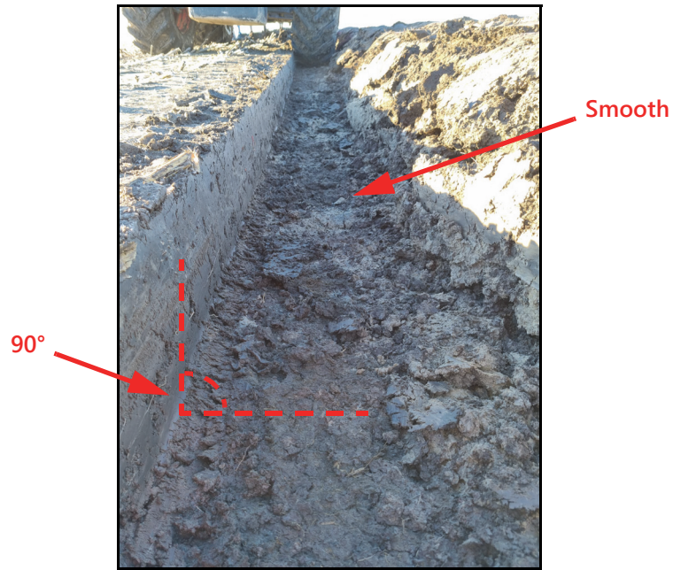
FIGURE 1. Proper Plough Leveling
