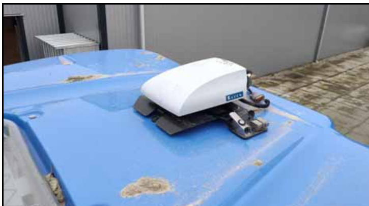
FIGURE 4. RS1 Mounted and Cable Connected
