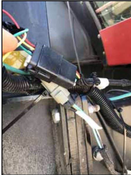
FIGURE 14. 12-Pin Aux Sensor Connected to VSN Cable
