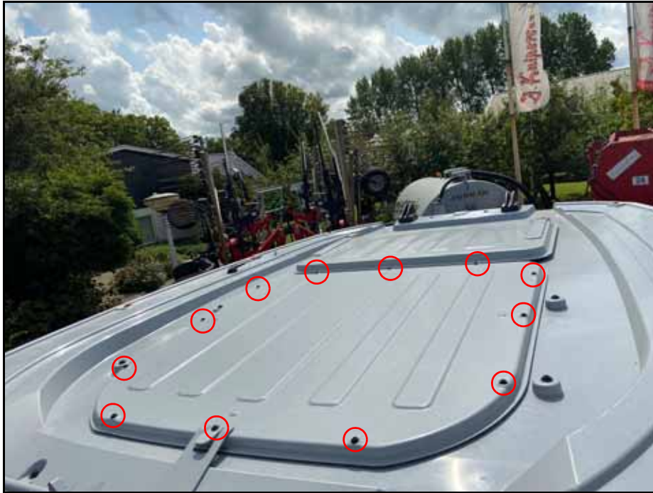
FIGURE 5. Roof Access Panel
