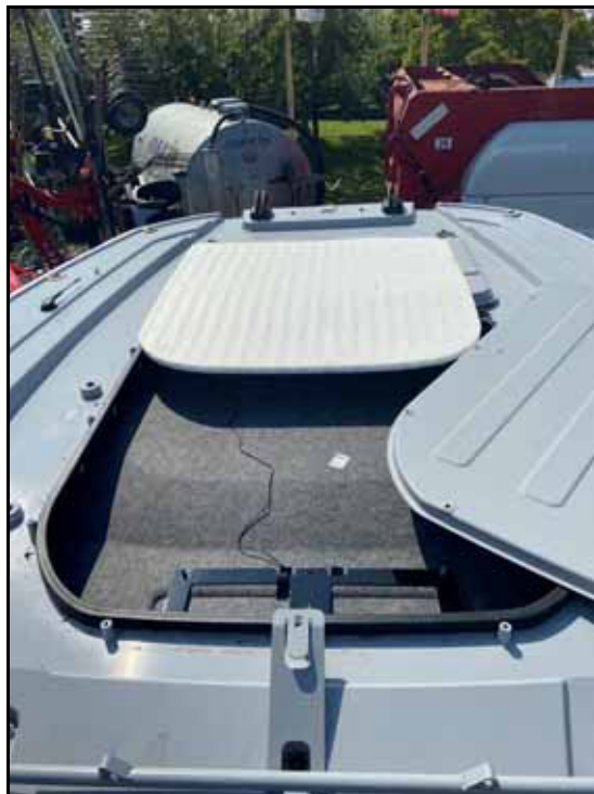
FIGURE 6. Roof Access Panel and Insulation Removed
