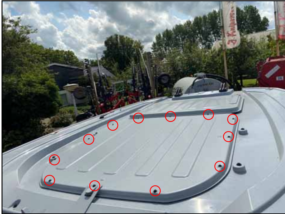
FIGURE 7. Roof Access Panel
