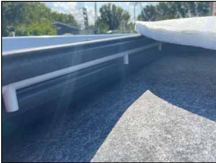
FIGURE 9. Space Between Roof Panel and Ceiling
