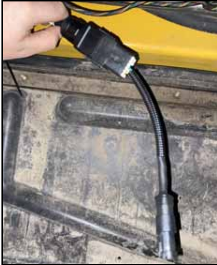
FIGURE 15. 12-Pin-to-3-Pin Terminator Cable Removed
