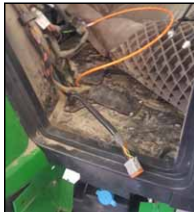
FIGURE 2. Cable Routed through Cabin Floor
