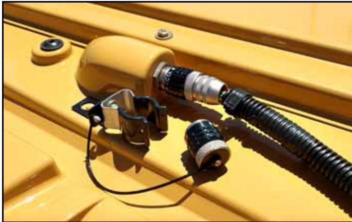
FIGURE 8. Completed Cable Connection
