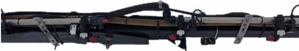
FIGURE 4. Outer Boom Cable Section Installed
