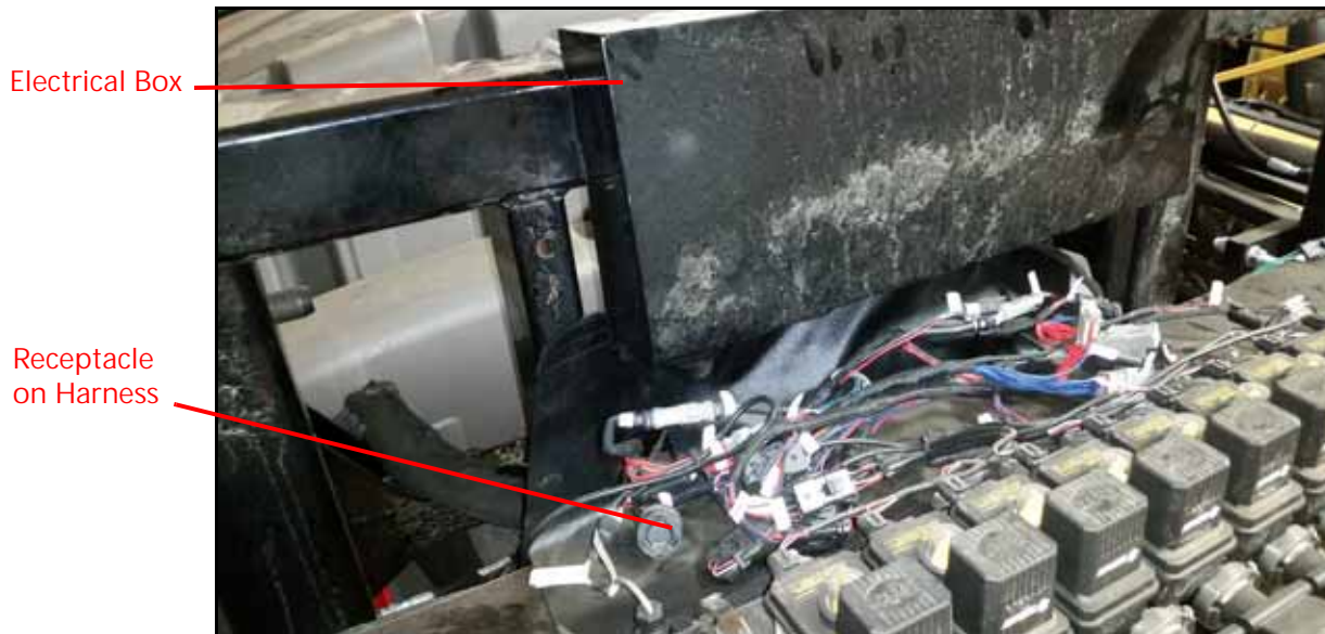
FIGURE 12. Harness Under Electrical Box
