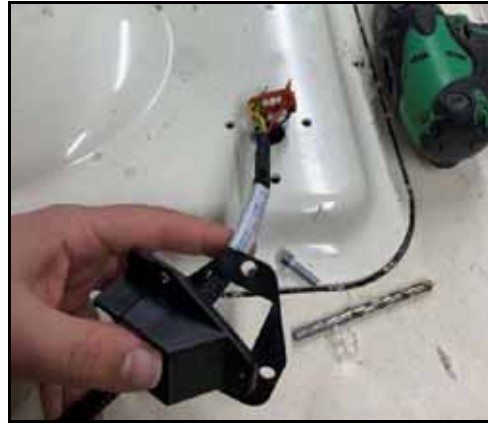
FIGURE 10. Cable Routed Through Roof Gland and Center Hole
