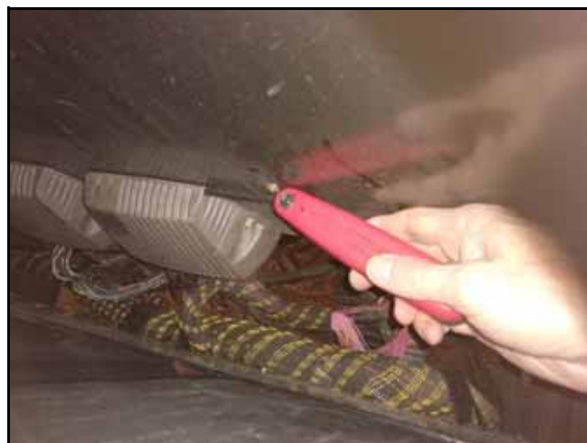
FIGURE 3. Brown Plastic Box Near RCM - Sprayer Mounting Location
