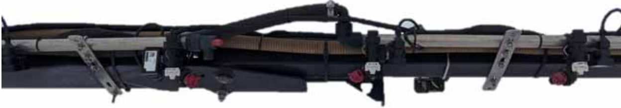
FIGURE 4. Outer Boom Cable Section Installed
