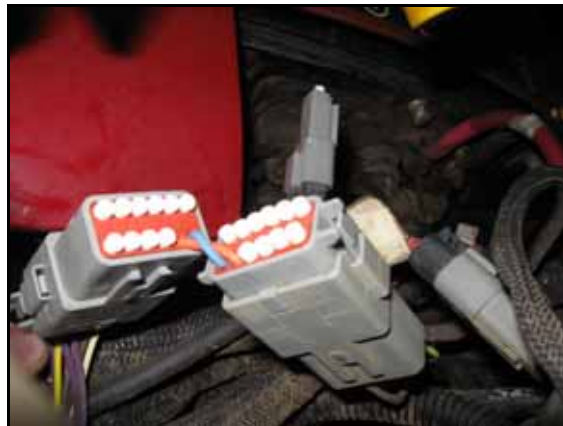
FIGURE 15. Fence Row Adapter Cable Installed
