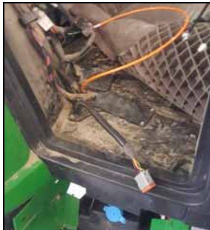
FIGURE 7. Cable Routed through Cab Floor
