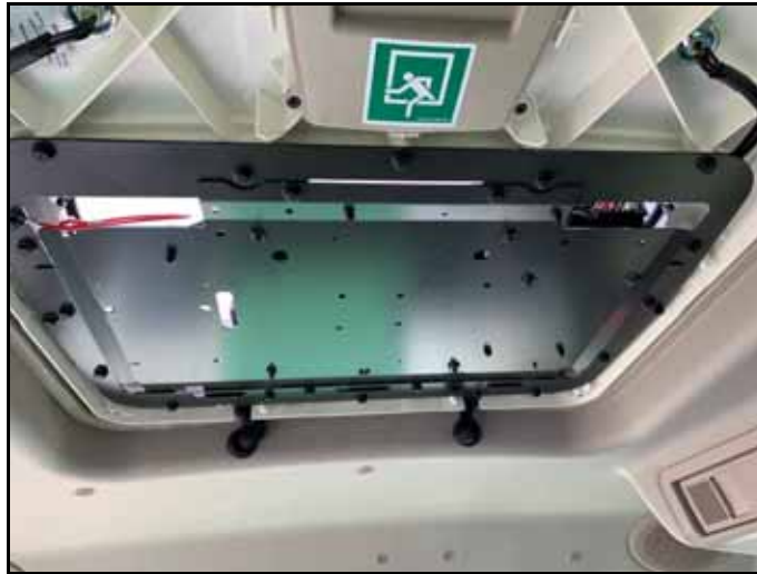
FIGURE 3. Roof Hatch Lining Removed
