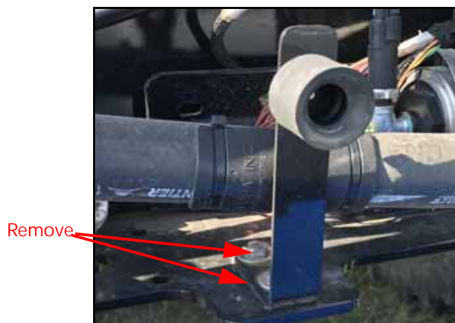
FIGURE 2. Two Bolts to be Removed
