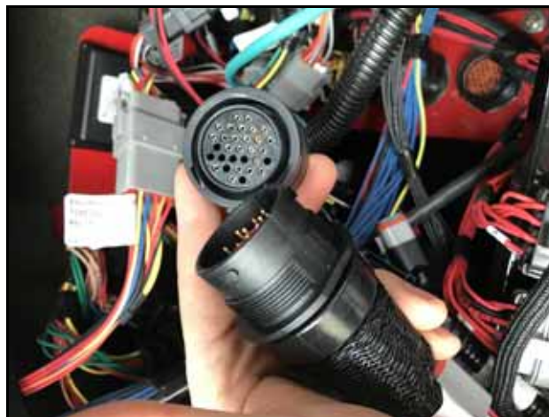
FIGURE 14. Mating Cable Connected to C9 Cable Connector
