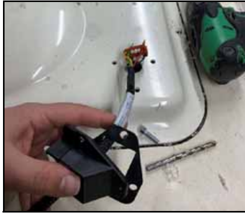
FIGURE 3. Cable Routed Through Roof Gland and Center Hole
