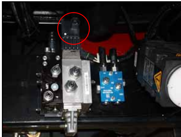
FIGURE 9. VALVE Harness Cable Installation Location
