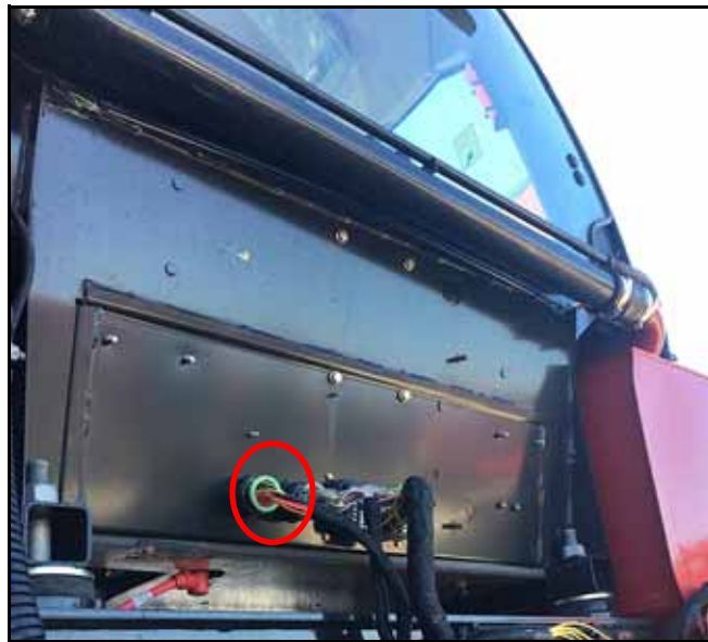
FIGURE 16. SC1 Tee Cable Connected to Machine's Bulkhead
