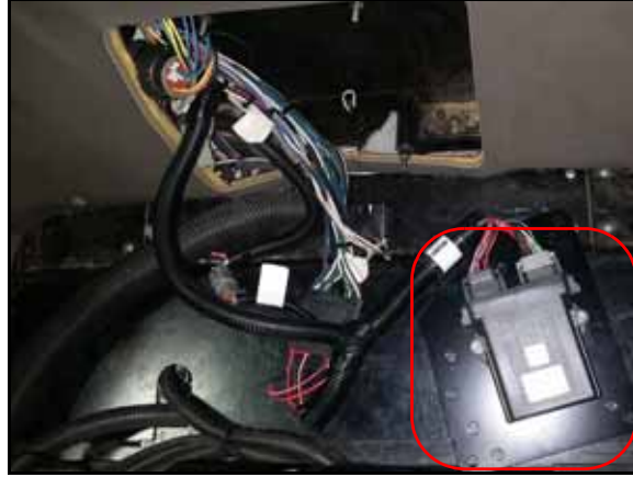
FIGURE 12. HDU Installed on HDU Mounting Bracket
