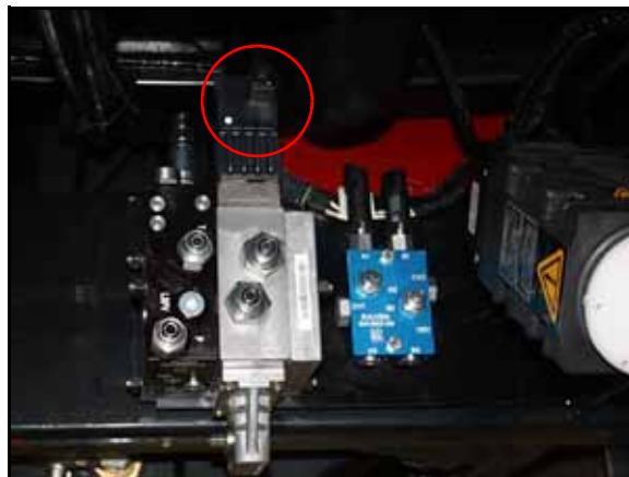
FIGURE 15. VALVE Harness Cable Installation Location
