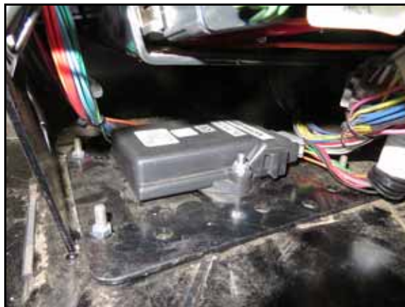
FIGURE 3. Node and Bracket Secured to Floor Studs
