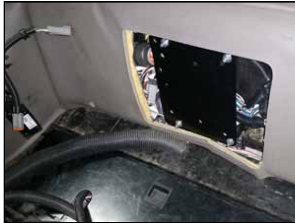
FIGURE 11. HDU Mounting Bracket Installed
