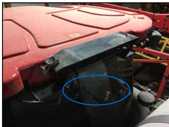
FIGURE 2. Existing GPS Receiver Cable
