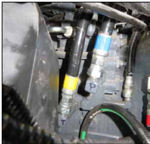
FIGURE 14. Pressure and Tank Hoses
