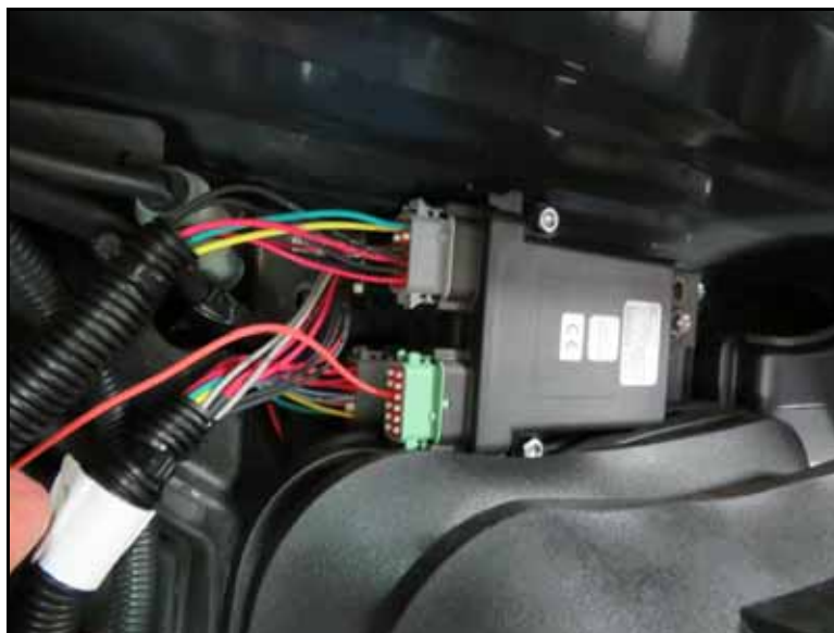
FIGURE 9. TC1 and HDU Cable Connection
