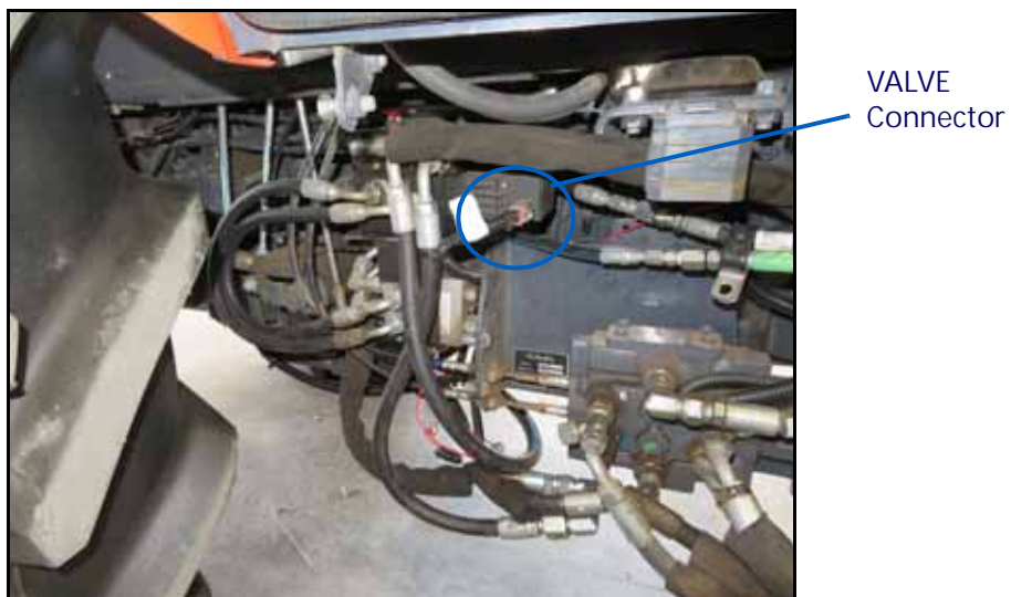
FIGURE 17. Valve Harness Connected to the Hydraulic Steering Valve
