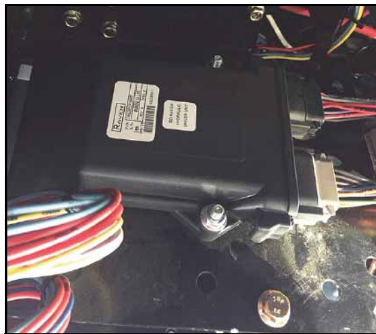
FIGURE 5. 12-Pin HDU Cables Connected
