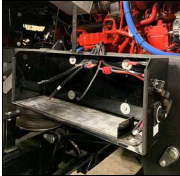
FIGURE 4. Installed Rear Vertical Support Bracket
