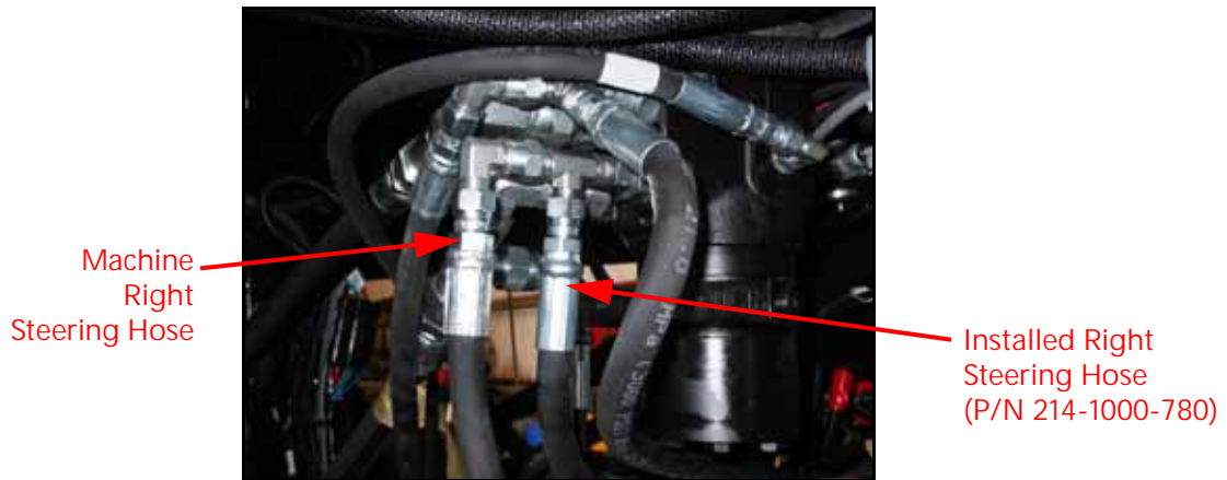
FIGURE 9. Right Steering Hose Installed on Steering Orbital
