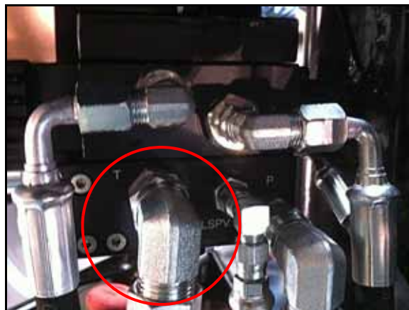
FIGURE 14. Tank Hose Installed on Steering Valve
