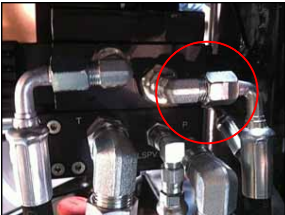
FIGURE 10. Right Steering Hose Installed on Steering Valve
