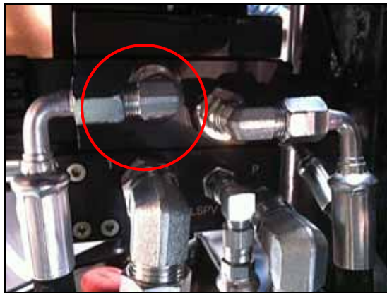
FIGURE 7. Left Steering Hose Installed on Steering Valve
