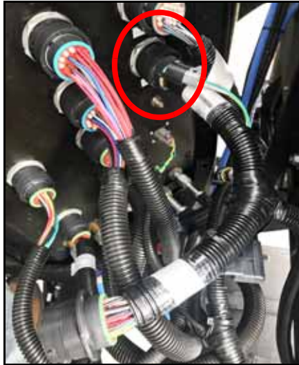
FIGURE 17. RS1 Tee Cable Connected to Raven Bulkhead Port
