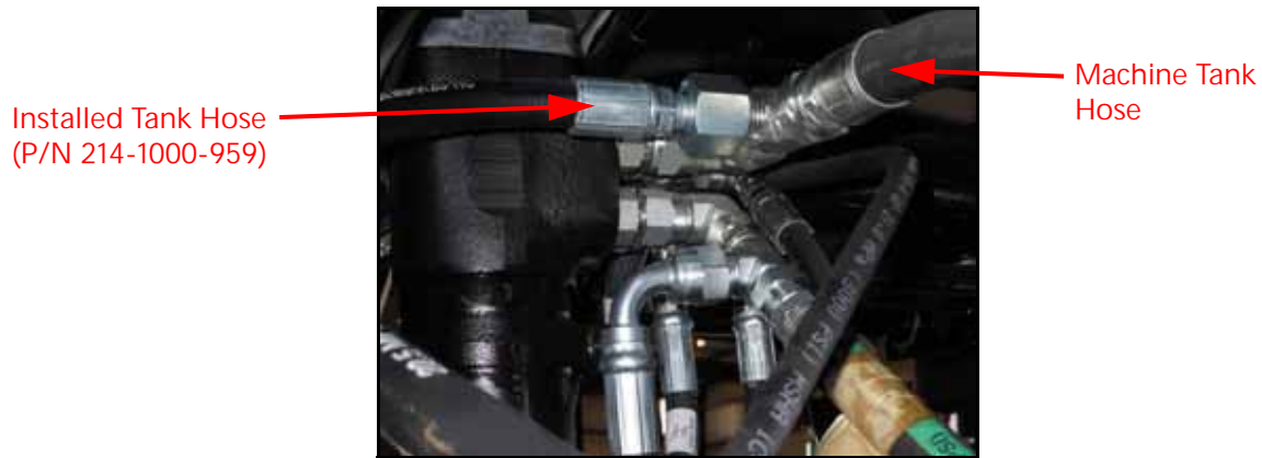
FIGURE 13. Tank Hose Installed on Steering Orbital
