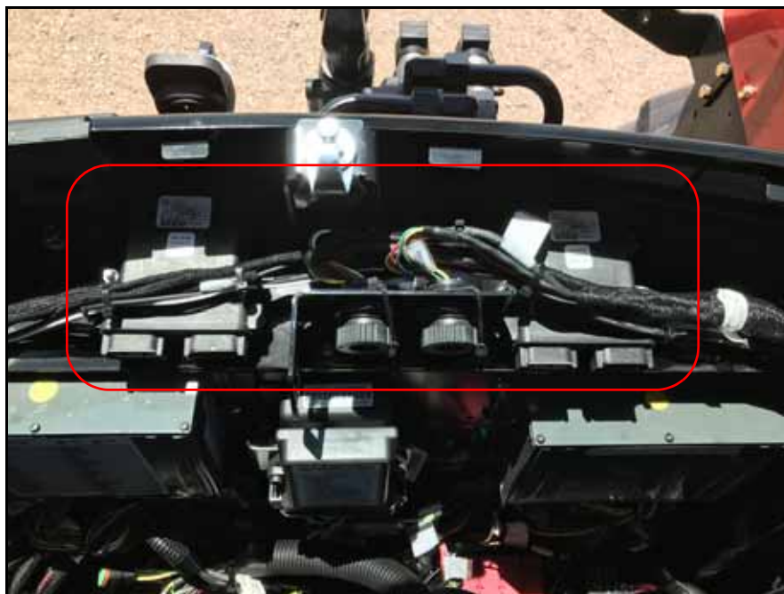
FIGURE 3. Node Mounting Location After Installation
