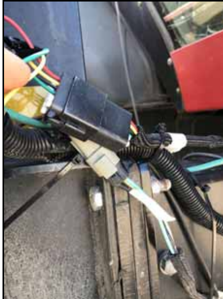
FIGURE 20. 12-Pin Aux Sensor Connected to VSN Cable
