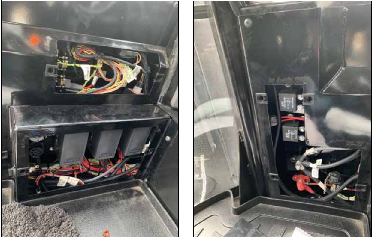
FIGURE 9. Interior Access Panels Removed
