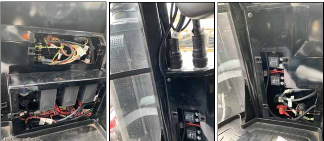
FIGURE 10. Interior Cable Routing
