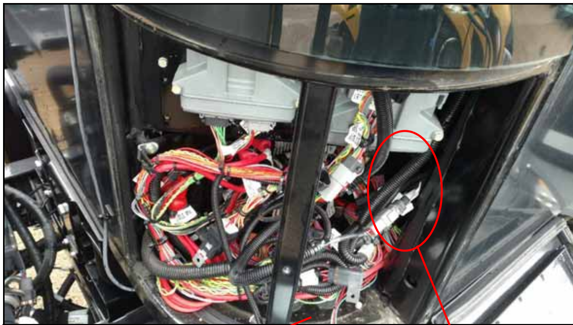
FIGURE 9. Exterior Access Panel Removed
