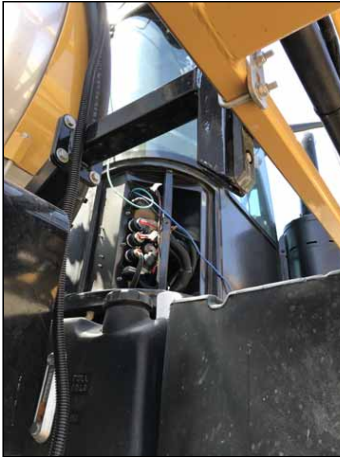
FIGURE 8. Exterior Cab Access Panel Removed from Right Rear
