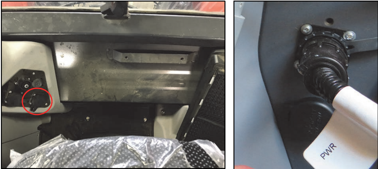
FIGURE 4. Power Terminal Location
