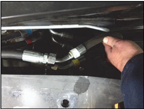
FIGURE 17. Hydraulic Hose Installed on Right Steering Hose
