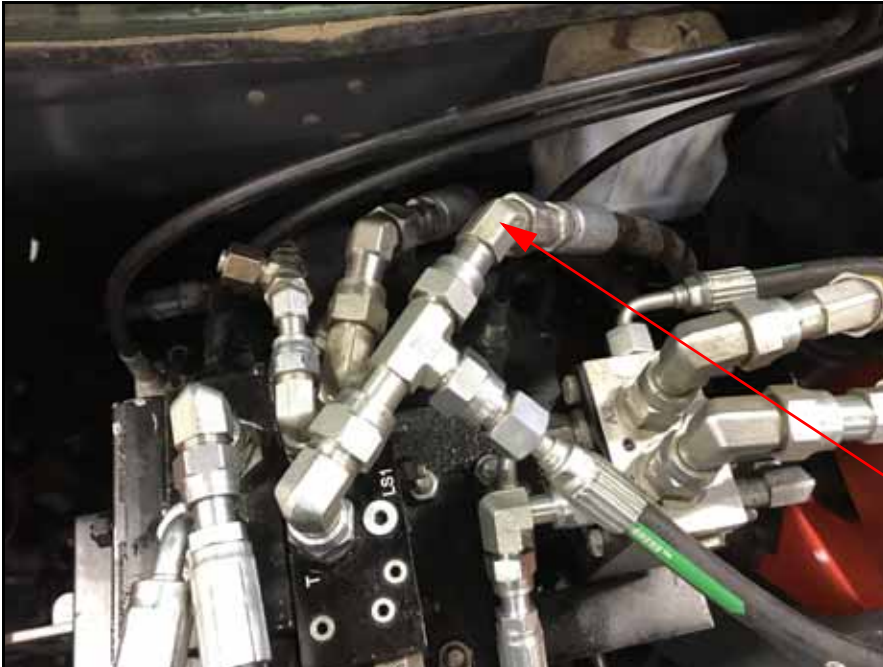
FIGURE 32. Tank Hose Installed on the Hydraulic Steering Valve
