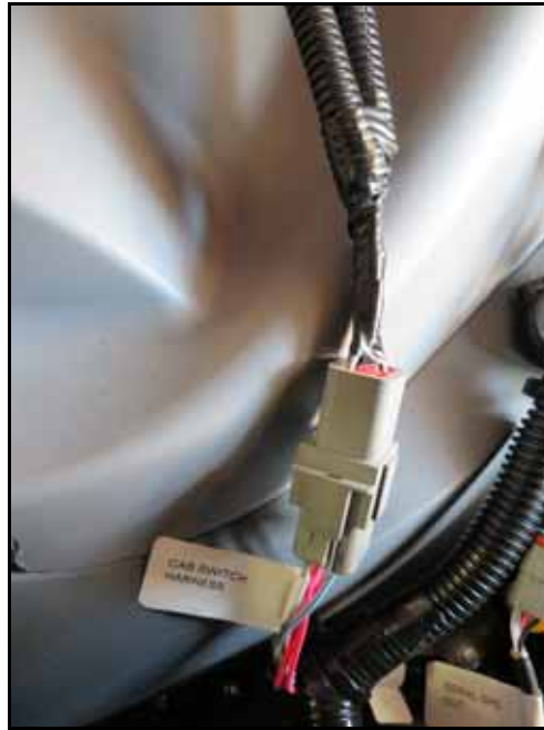
FIGURE 6. Cab Switch Harness Connection
