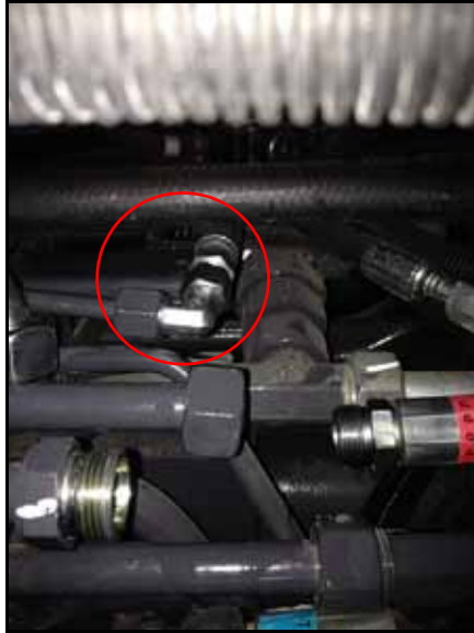
FIGURE 25. Hydraulic Hose Installed on Steel Load Sense Line
