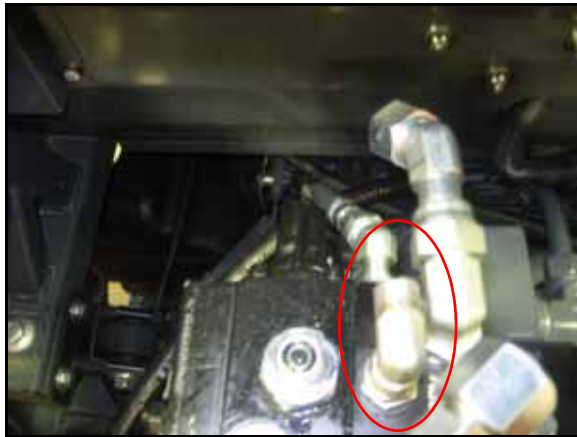
FIGURE 26. LSPV Hose Installed on Hydraulic Steering Valve
