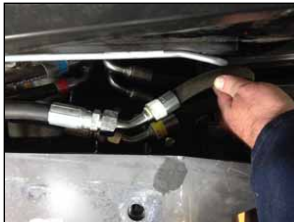
FIGURE 12. Hydraulic Hose Installed on Left Steering Hose
