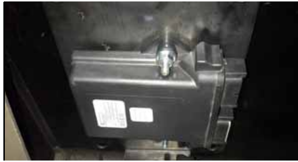
FIGURE 15. HDU Mounting Bracket Installed
