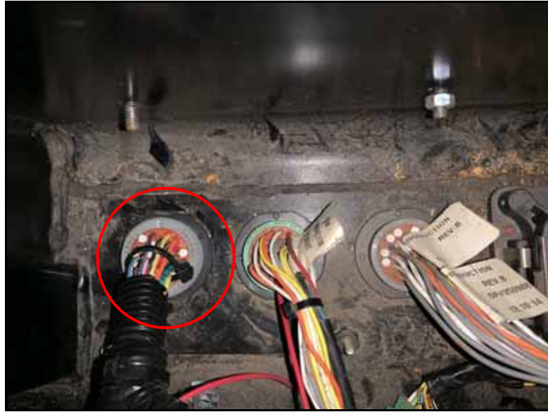
FIGURE 5. Existing Machine XB-7 Bulkhead Connection
