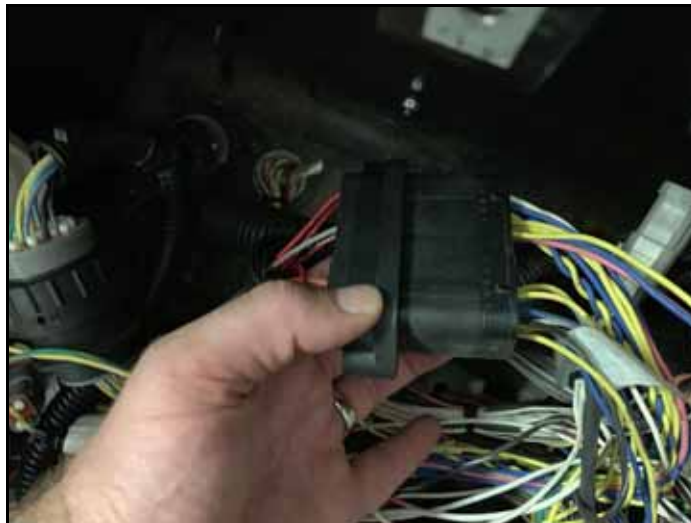
FIGURE 6. Existing Machine XB-7 Bulkhead Connection
