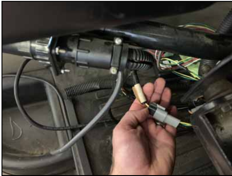
FIGURE 7. HDU Cable Connected
