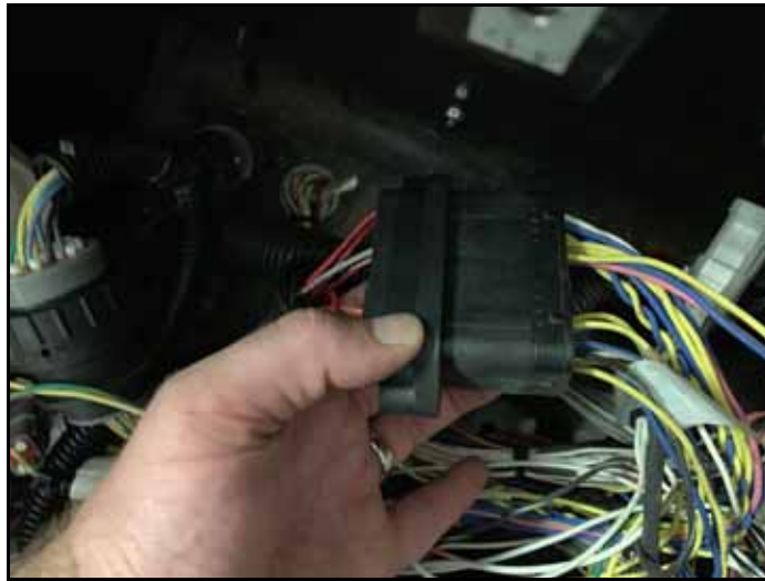
FIGURE 5. Existing Machine XB-7 Bulkhead Connection
