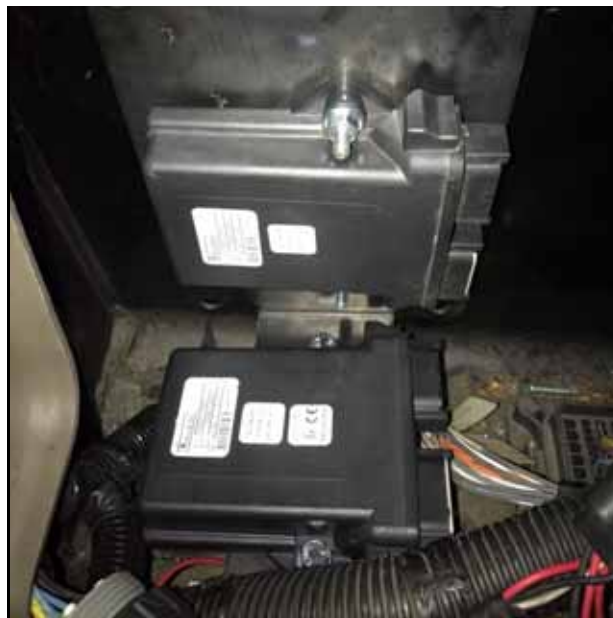
FIGURE 14. HDU Mounting Bracket Installed
