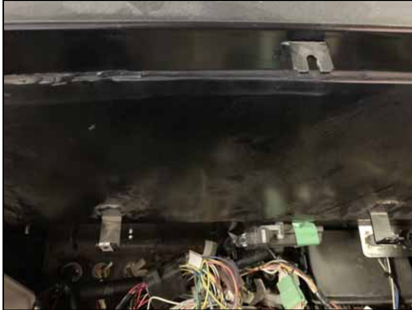
FIGURE 3. Access Panel to be Removed
